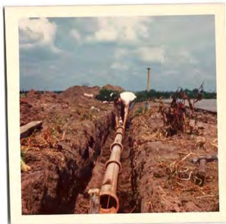
Laying drainage channel.
