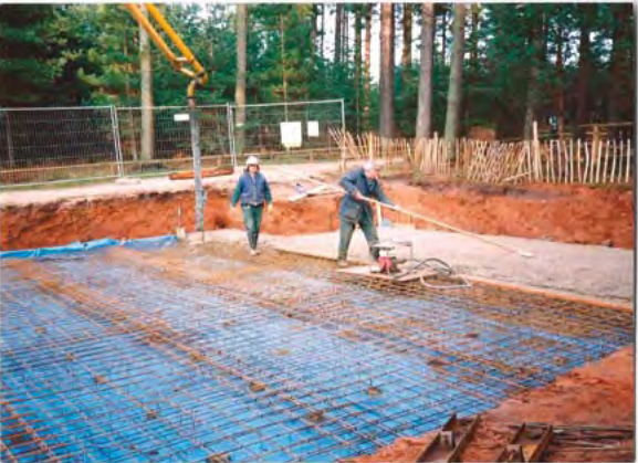
The foundations-pump 'elephant's trunk'
